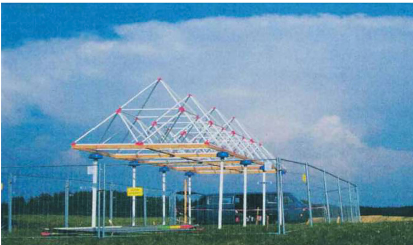
Figure 1. An early photograph of a ground-based ioniser installation. Its location is uncertain, but on the basis of the accompanying documentation, it is likely that the photograph was taken in Russia before 1999.
